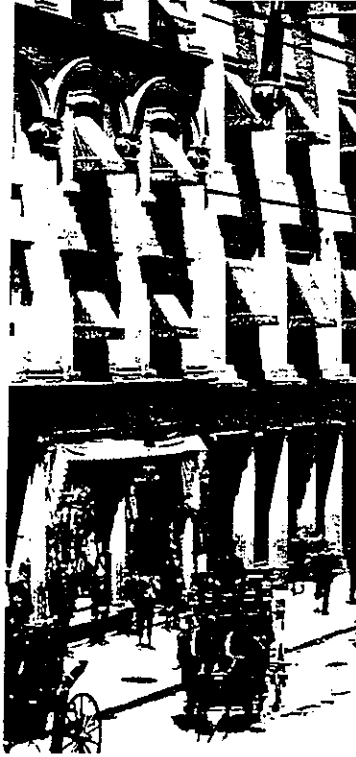
2. Awnings on a 19th century commercial building
