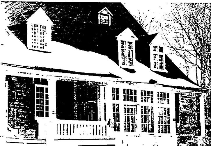
1. Sunroom made by enclosing a veranda: These sunrooms are usually made out of wood and built directly onto the gallery which is sometimes reinforced.
